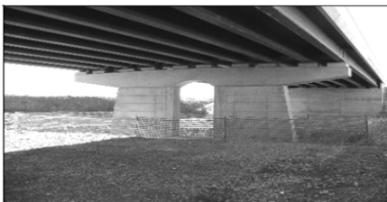
Fig 1.5: Bourg-lès-Valence Bridge, France, 2004
